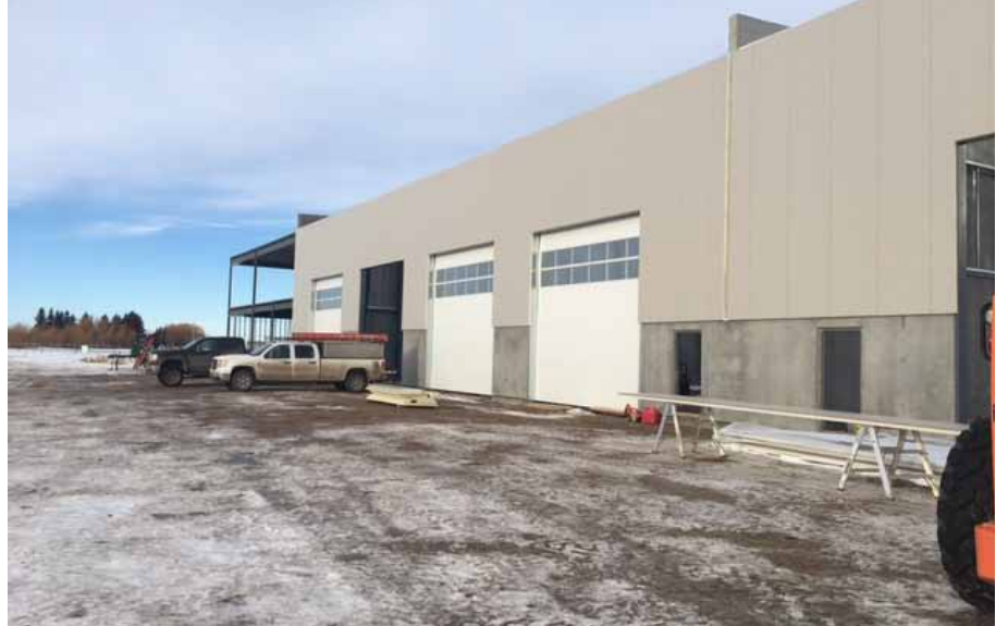
The new Public Works Facility has 'Wet' ponds which are required by the Province of Alberta as set out in Stormwater Management Guidelines, to handle storm water runoff.
