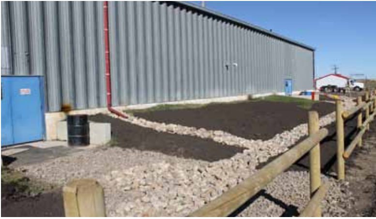
Fixing a Byemoor drainage problem.
