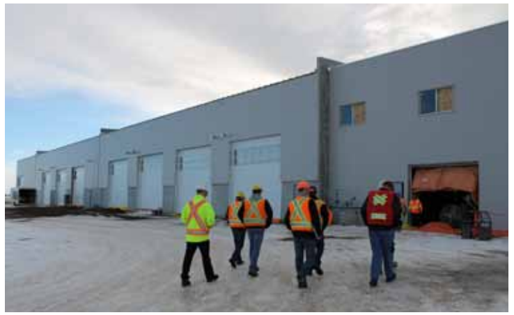
The new Public Works Facility under construction.
