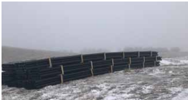
Water pipe ready for installation to White Sands.
