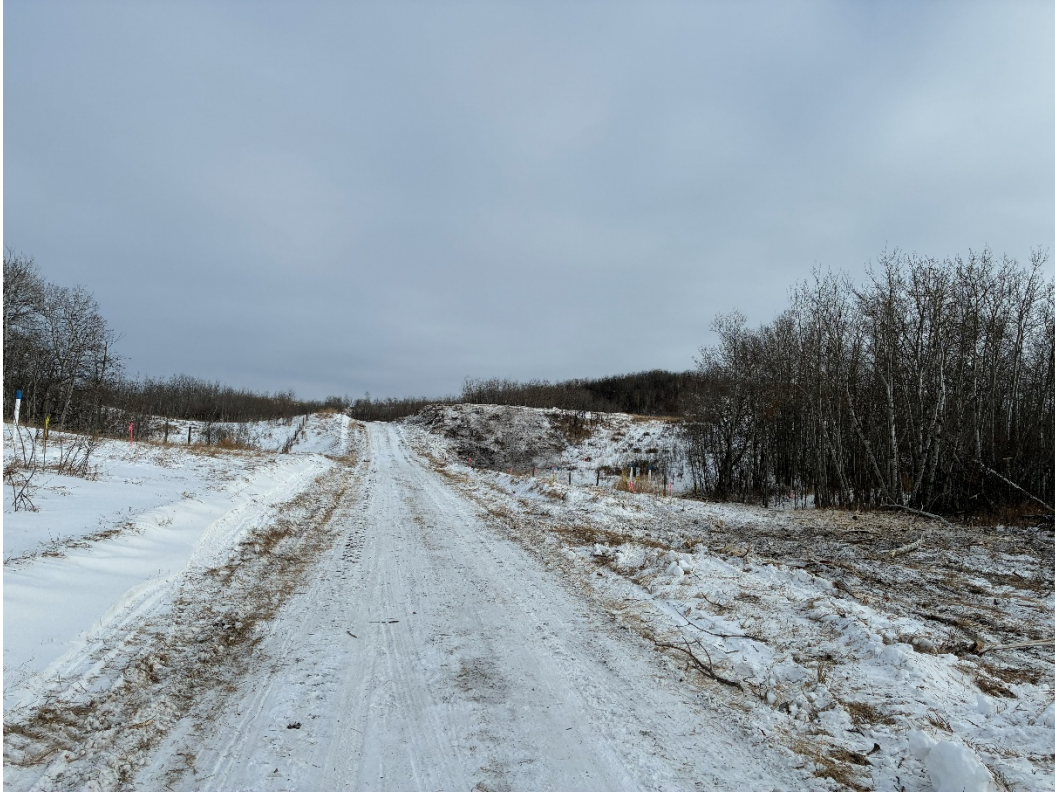
PW Figure 0.09. Rge Rd 34-4 - Back Road Fenceline Dozer Brushing
