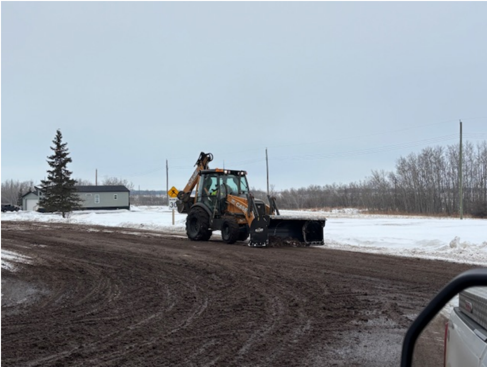
PW Figure 0.02. Botha Street Cleaning
